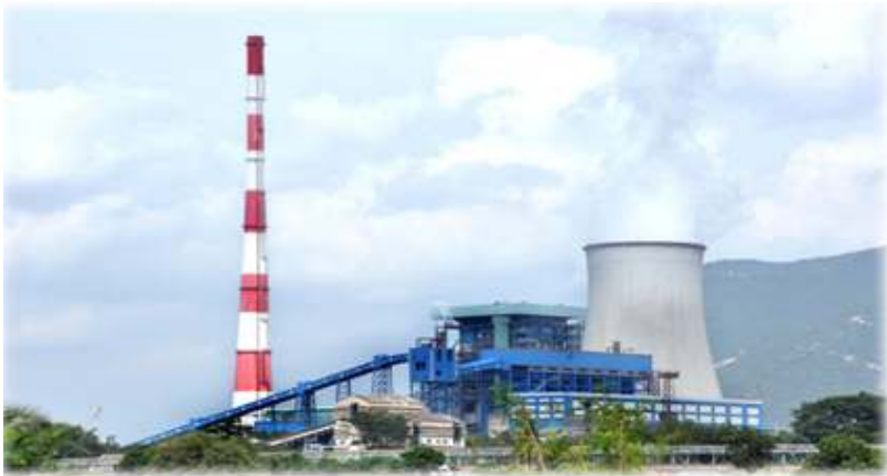
Mettur Thermal Power Station – II
