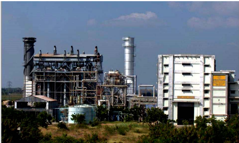
Thirumakottai Gas Turbine Power Station
